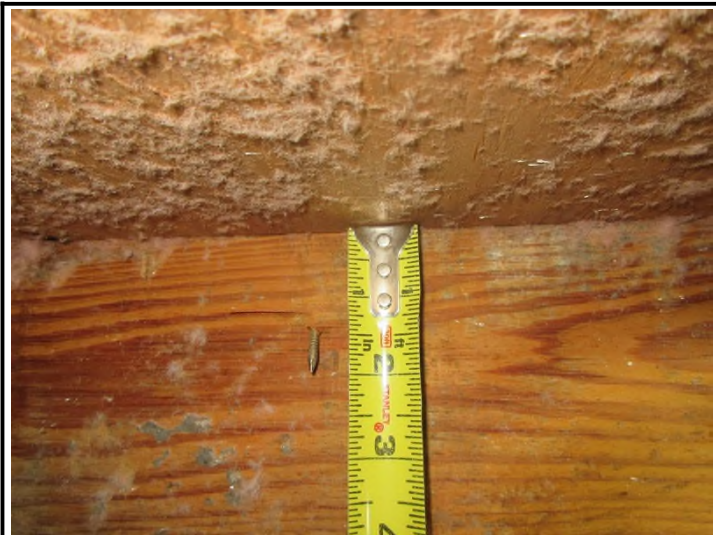
8d nails spaced 6" in the field
