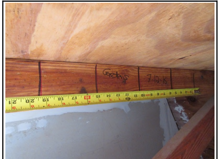
8d nails spaced 6" in the field
