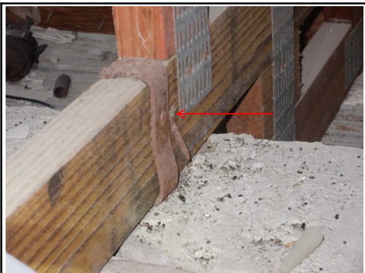
Metal straps with 1 nail on the front side
